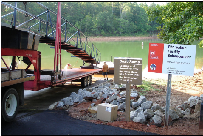
"Custom" dock & gangway being installed at 18 Mile Creek
