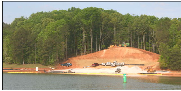
Megaramp construction at Tugaloo State Park near Lavonia
