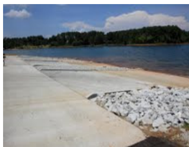
Six new ramps at Gum Branch
