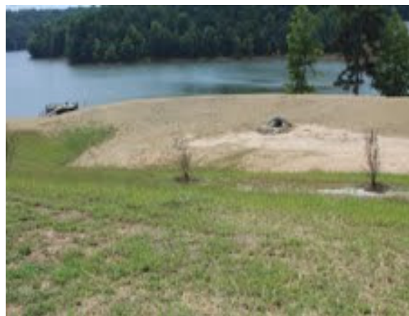
Tugaloo Retention Pond
