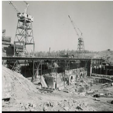
April 16, 1959. Concrete bucket being picked up by whirley to be lowered into forms. 20 ton American Revolver Crane on 70 foot Gantry Crane, 150
