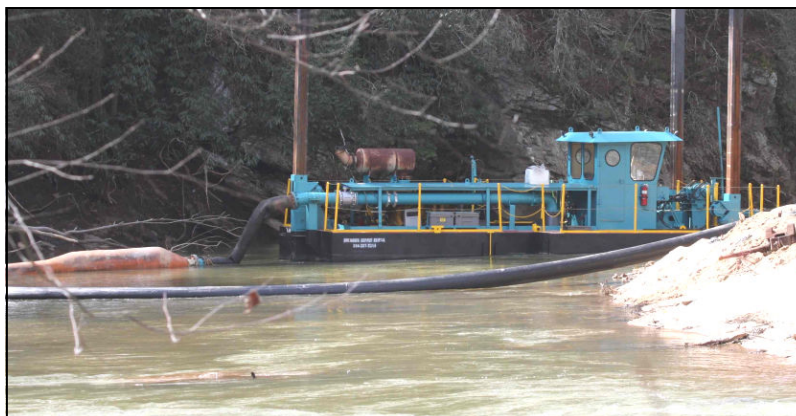
Workers begin removal of two dams on Twelve Mile River
