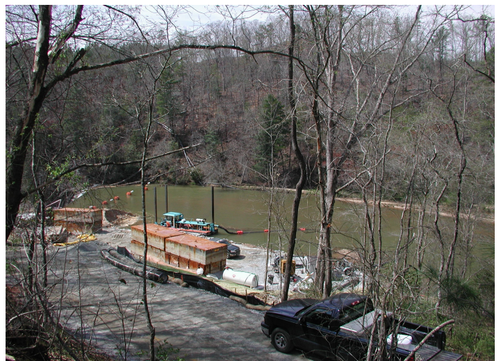
Dredge in Twelve Mile River
