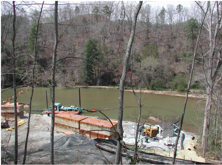
Dredge in Twelve Mile River
