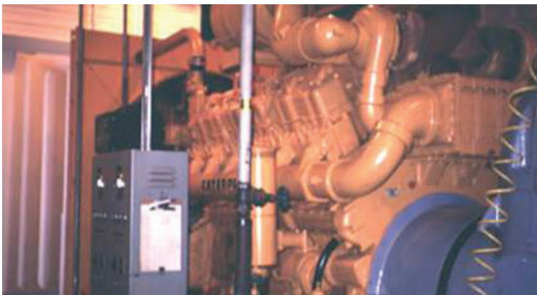
One of the Diesel engine pumps
