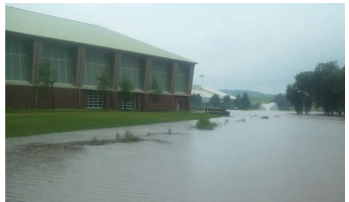
New indoor football training facility
