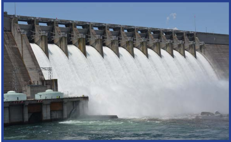
All spillways open for testing
